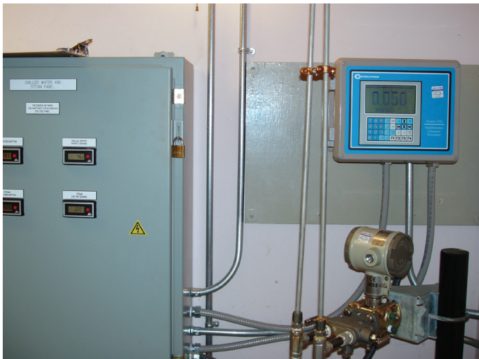
Typical customer metering system installation.
