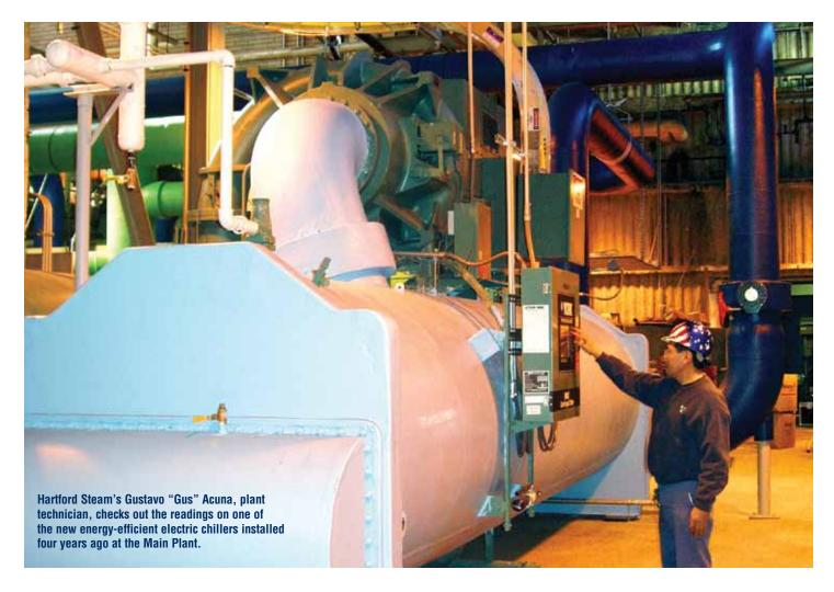
emissions. The new chillers replaced a 4,500-ton steamdriven chiller, which now increases our system reliability as a backup unit.
